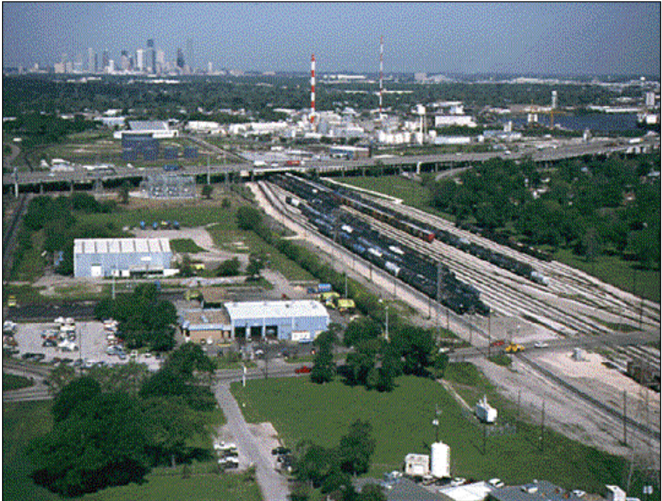
Overall Site View of HRM 01 Monitor Location
